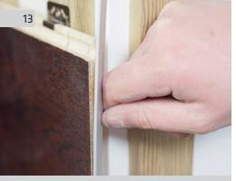
Then glue in an aluminium flat bar, for example, at this point, which serves as both decoration and protection on the sharp trimmed edge. Aluminium or wooden angle bars can be used instead.
