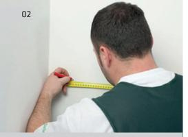
Mark the places where the wooden construction floats, with a cross-section measuring at least 18mm x 50mm, are to be attached. Attach the first float a maximum of 10cm from the internal or external corner.
