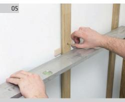
The floats must form a single plane. Check this by using a spirit level applied over a width of at least 3 floats. If necessary use plywood or other material to level the structure.
